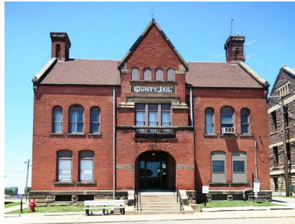
Figure 2.2 Historic Perry County Jail
